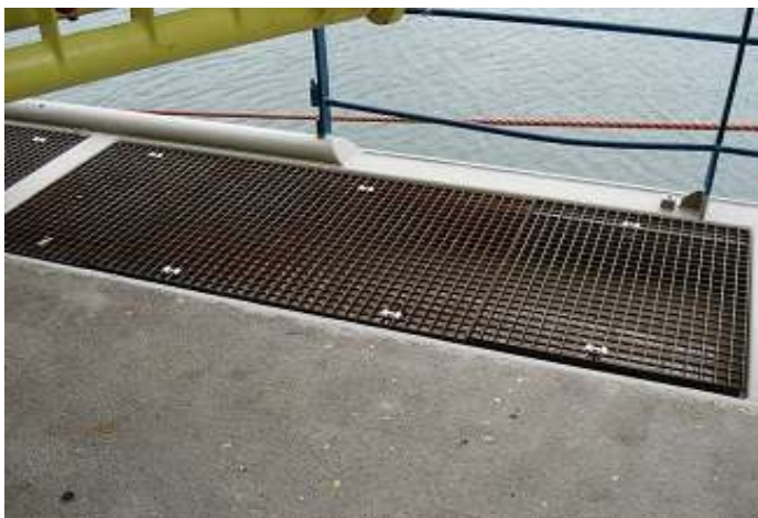
Before, the corroded steel gratings
