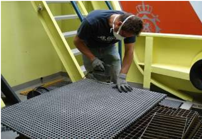
Cutting panels with Jigsaw
