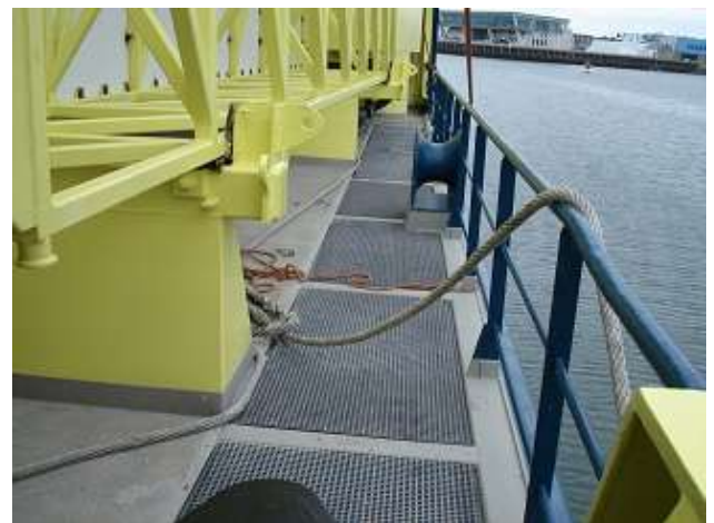
After, the new Swiss Solutions Gratings
