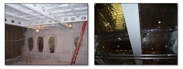
Mascoat Marine-DTM applied to the outside wall of the vessel and framing supports to combat condensation/sweating. The coating is normally applied to 40-80 mils (1.0-2.0 mm) in a series of coats. By applying the coating to the side walls, stiffeners, overheads and shells of the vessel, protection is given as well as reducing radiant heat gain.
