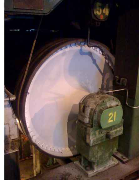
Figure 3 - Dryer can coated with Mascoat Industrial-DTI
