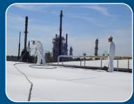
Mascoat Industrial-HR is a thermal insulating coating with highly reflective particles that is formulated to provide radiant heat gain protection for tanks, vessels, and other facility surfaces that are affected by solar loading. The coating can effectively protect internal contents from rising above desired temperatures. By using the coating, customers can efficiently stabilize processes, protect personnel, and consistently maintain product levels.
