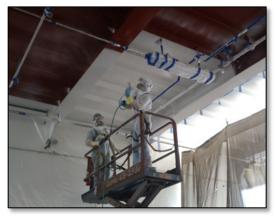
Over an epoxy primer, 120 mils of DTM was applied to the vessels. The short application time and easy process was a welcomed benefit. The vessels haven't experienced any corrosion or condensation issues since application and the insulated areas are much more bearable and cooler.
