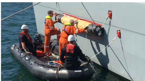
Installation of Polar Plaster
