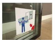
Example of an A60 CONTRAFLAM MARINE glass. Red corners shows how the glass need to be installed (which side up and down) and the pink label shows with text which side must be inside.
