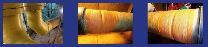
**RMN and WENCON** are also involved in many Exhaust gas scrubber repairs. We developed a repair method for corrosion pittings in the different areas of the scrubber system. Due to the extreme harsh environment inside the scrubbers with a very low Ph value we use the Wencon Hi-Temp and Wencon Ceramic Products to withstand the temperatures and Ph values.
