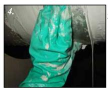
3+4. Larger holes are easily being repaired by glueing a thin steel plate in combination with reinforcement tape. The final results will resist a relativ high pressure.
