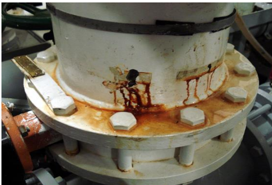
Tercoo® result on an old steel pipe to clean the surface and make a good roughness for a repair job. Job done with the Tercoo® Single disc and Trio disc on a hand drilling machine.
