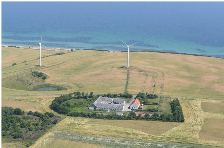
Siemens Bonus 500 wind turbine.
